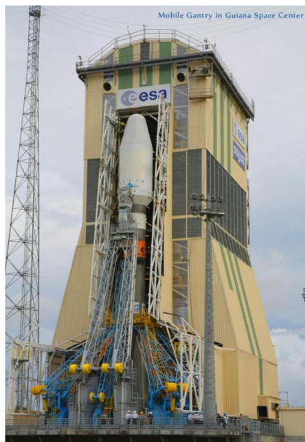
Mobile Gantry in GSC
